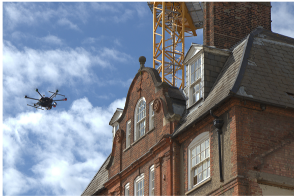
Inspecting large-scale structures
